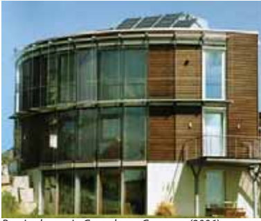
Passive house in Guenzburg, Germany (2006). Source: UCD Energy Research Group.
