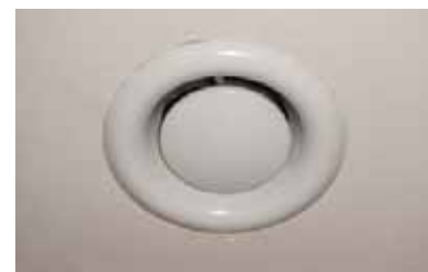
Ceiling air supply vent. Source: MosArt Architecture.
